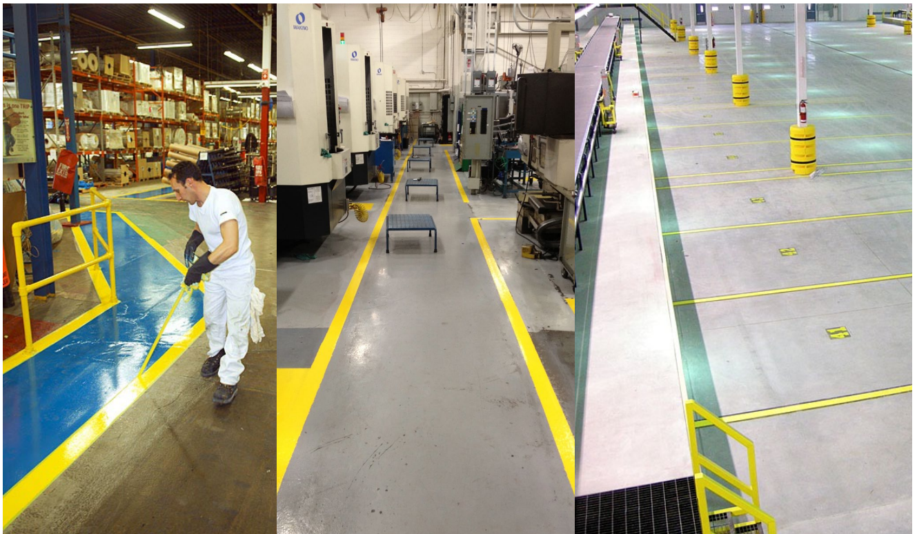
Left: Blue walkway with applied yellow safety lines in Sonoco manufacturing facility. Centre: Epoxy safety lines designating walkway areas in Exco facility. Right: FedEx warehouse yellow epoxy walkway safety and truck parking lines.
