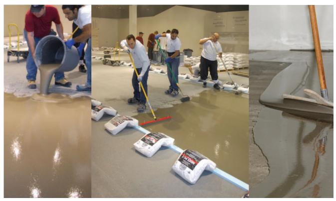
Left: 3/8" Polished Concrete Topping being poured on floor at North Face Store, Yorkdale location.
