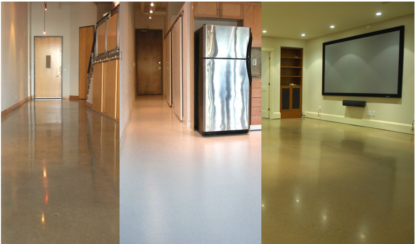
Left: Polished concrete floor in downtown loft. Centre: Apartment floor with White epoxy and white urethane coating. Right: Apartment with Clear Epoxy with Clear Satin Urethane.
